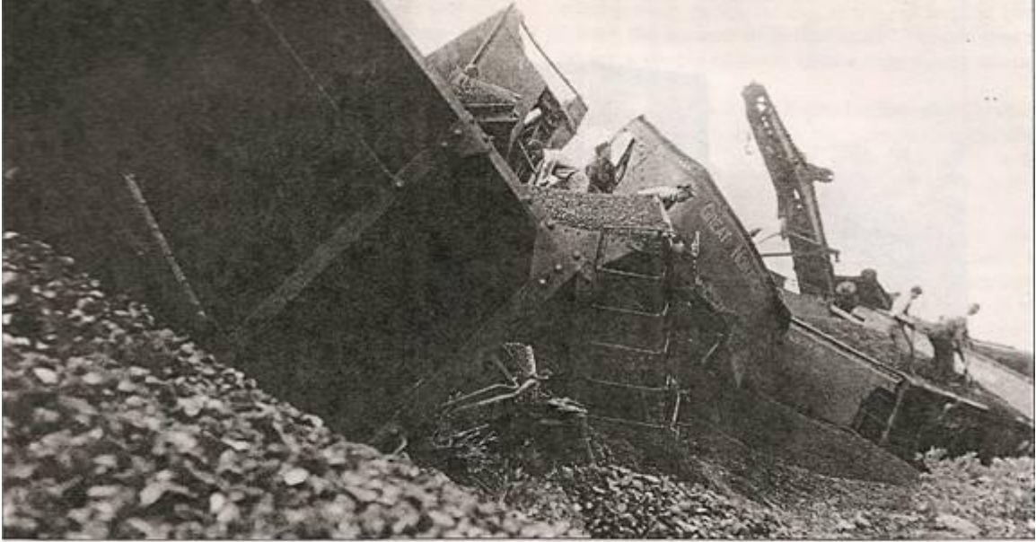
Accidents are never pretty scenes, particularly when lives are lost as a result. This 1949 ore car train derailed caused the death of train engineer Steve Miller, buried under ore from the overturned ore cars.
